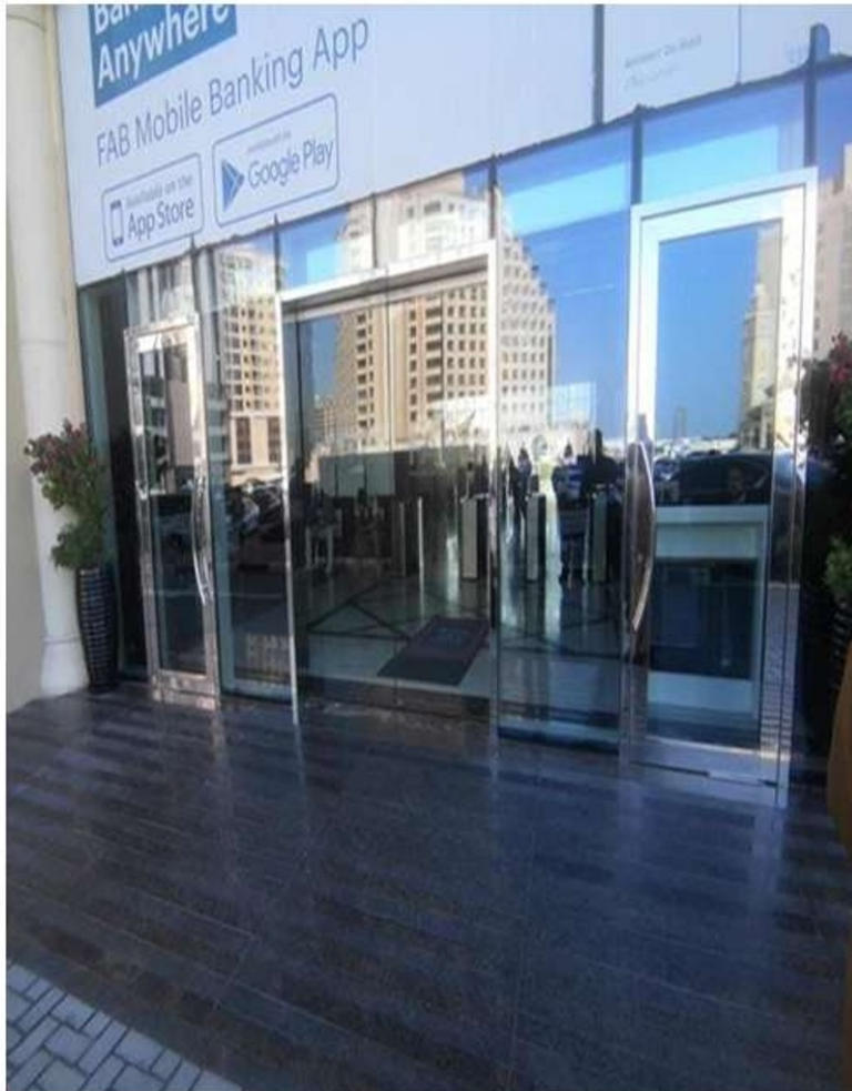
ELGM - Before and while working
