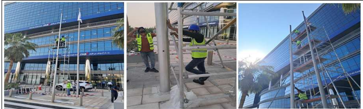
Work Completed Location: FAB – Al qurm, Abu Dhabi UAE
